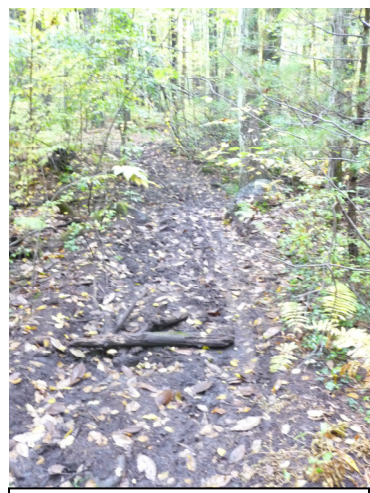
Rutted trail crossing over seasonal drainage.
